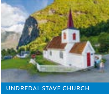
UNDREDAL STAVE CHURCH
